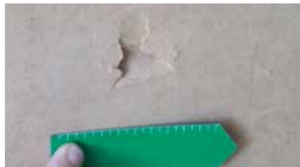
☰ Houten binnenbekleding: Kleine deuken
